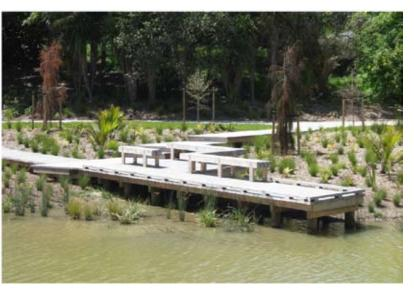
A boardwalk platform provides proximity to the wetland. Macrocarpa was used in place of treated pine or sustainable tropical hardwoods (in limited supply). Similar to other aspects of the project the boardwalk platform mirrored NSCC park standards for decks, but were a bespoke design. The vegetation around the boardwalk will grow to form cabbage tree groves and kahikatea swamp forest.
