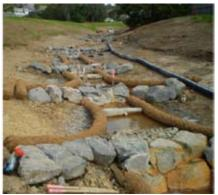
The Bayside project applied multiple 'bioengineering' approaches, including Filtrexx™ living walls in steep areas, dry-stone rock construction for weirs, coir (coco-
